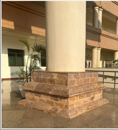
Image 3: Pillars base made out of laterite blocks in NISER Bhubaneswar
