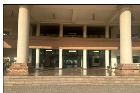
Image 3 : Pillar base made out of laterite blocks in NISER Bhubaneswar
